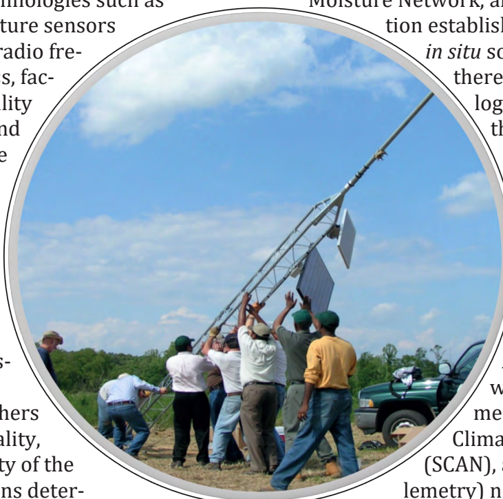
Raising a meteorological tower for a remote soil monitoring station
