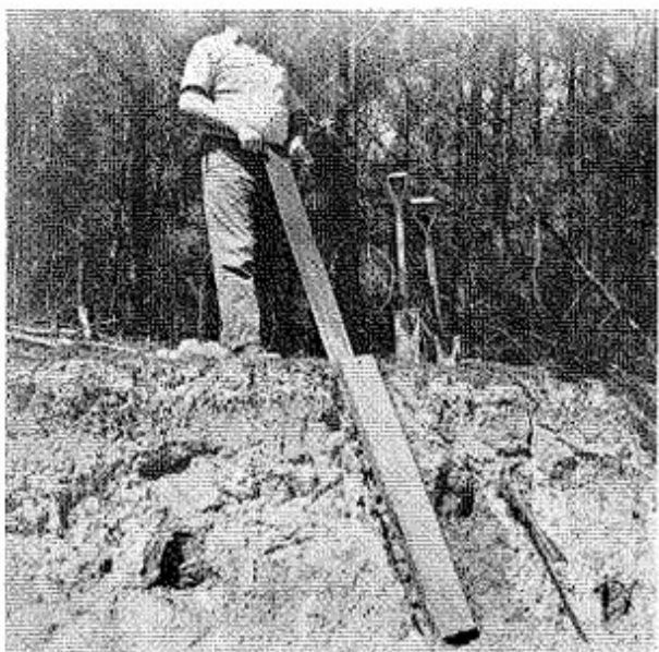
5. When moisture conditions are good, soil may be cut behind the frame with a special tool designed for the purpose.
